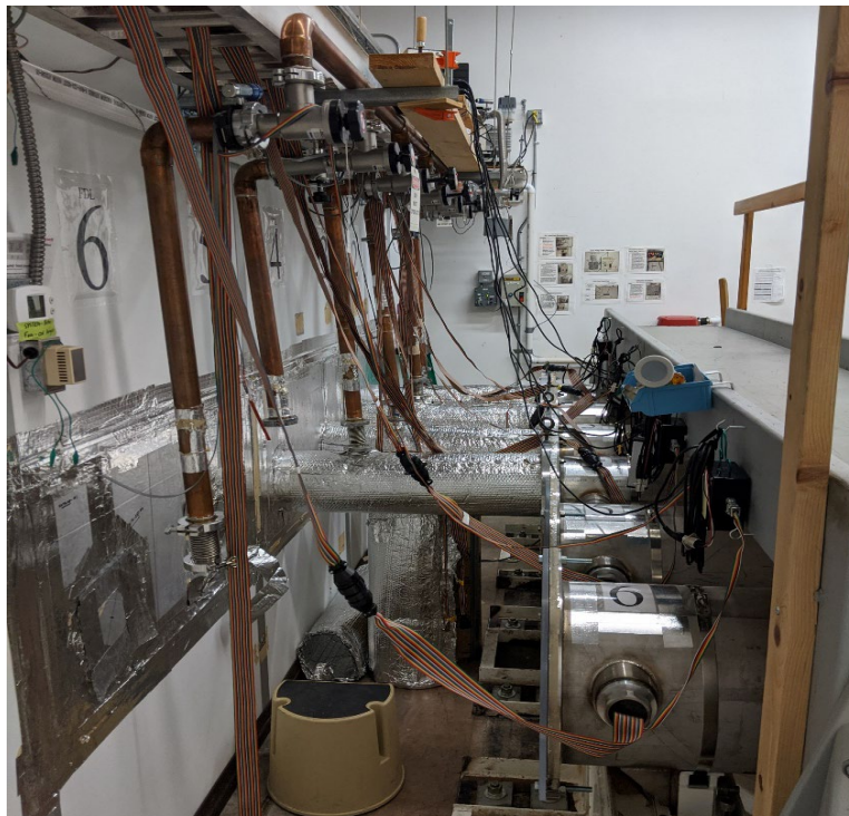
Figure 1: Where Pipes Connect to “snoot” on Original Vacuum Manifold at NPOI
